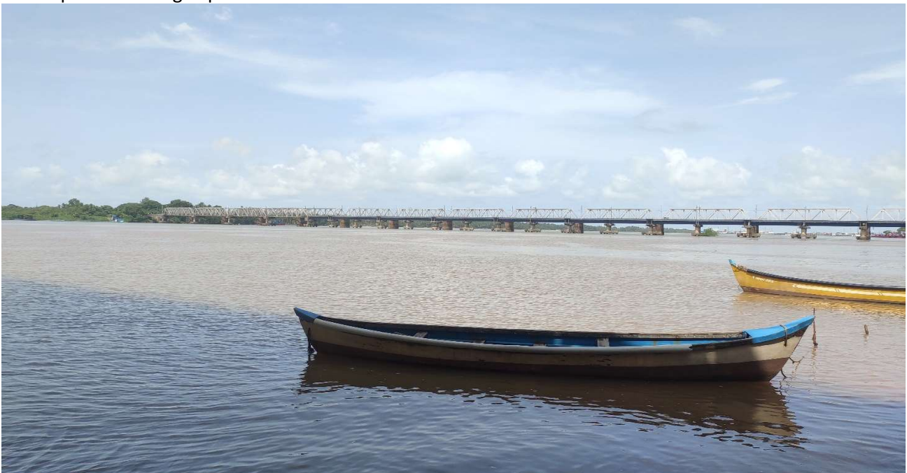
View of the Netravathi River and the bridge connecting Ullal and Mangalore
